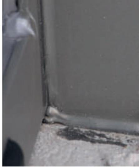
Figure 55.- Scellant incorrect (Source : ASEFAVE)
