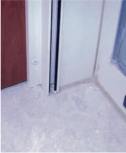
Figure 54.- Scellant correct (Source ASEFAVE, Association de fabricants de vitres)
